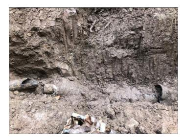
A break in the roof drain pipe was observed within the 8-inch diameter ductile iron pipe (DIP) section just inches before the hard connection to small diameter reinforced concrete pipes (RCP) that had settled multiple inches in two separate, short RCP pipe sections prior to tying into the underlying 54-inch RCP. The two sections of excavated broken and settled pipe sections are shown in the following photo.
